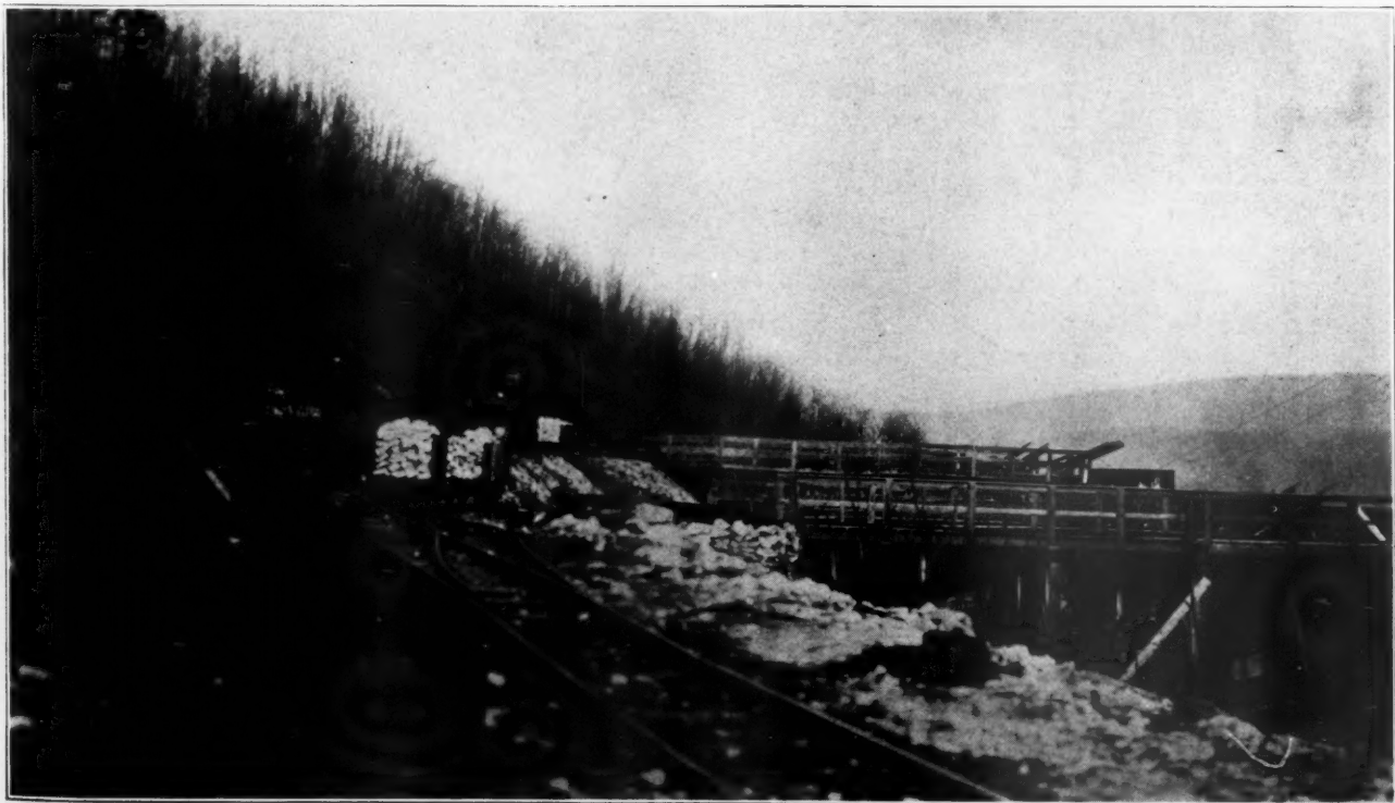
Tracks and Trestles to Top of Kilns
